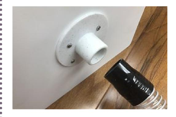
Secure the flange that came with the toilet to the inside, aligned with hole that was drilled.
