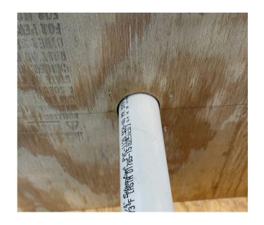
Take the piece of 1 1/4" PVC pipe (Not provided) and insert through the interior wall into the back of the shell vent.
