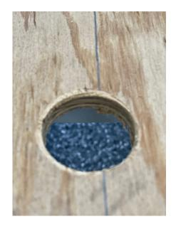
Using a 1 3/4" hole saw, drill hole through exterior wall.
