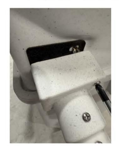
Alternare tightening the two screws until the housing is tight.
